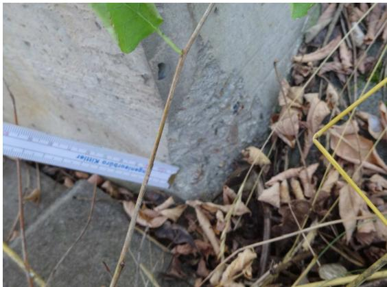
S15 BETONKANTE AM WDL ABGEPLATZT
